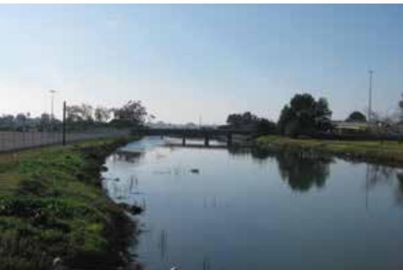
Damon Slough flood channel near Coliseum parking lot. Archival photo
