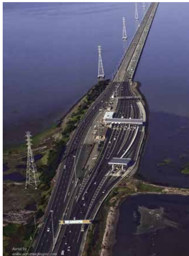
Vulnerable San Mateo Bridge landing. Photo aeroimaginginc@gmail.com
