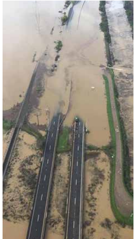
Flooding closed Highway 37 — a major North Bay east-west access route already plagued by congestion — during the winter of 2017. Photo courtesy Caltrans
